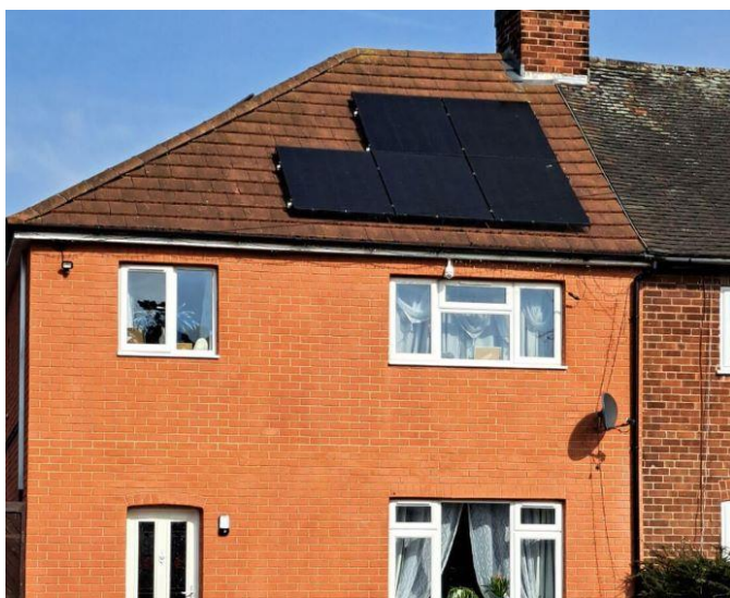
One of our tenanted properties benefitting from retrofitted energy efficient heating system upgrades
